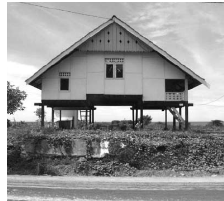
This house has been newly built after the tsunami in traditional Acenese style. With its steep stairs it is difficult for older people to enter.
